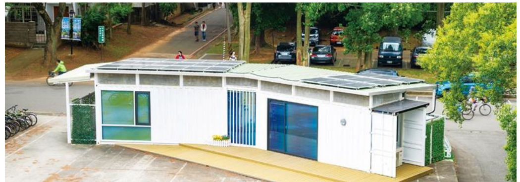
Figure 7. Microgrid system at National Central University, Taiwan.
