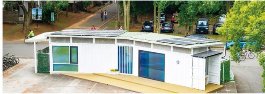
Figure 7. Microgrid system at National Central University, Taiwan.
